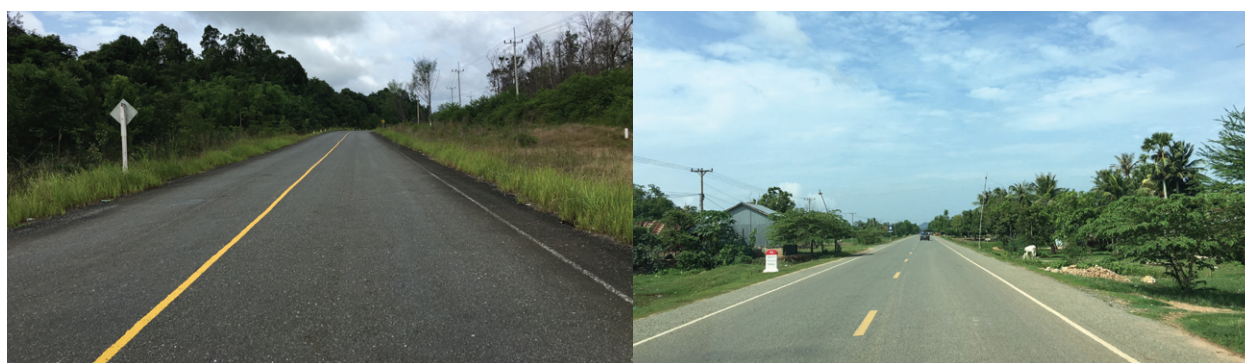
Left: Koh Kong-Sre Ambel. SEC-3 in Cambodia along NR No. 48. Right: Kampong Trach-Lork. Two lane double bituminous surface treatment road completed with an ADB loan in 2010.
