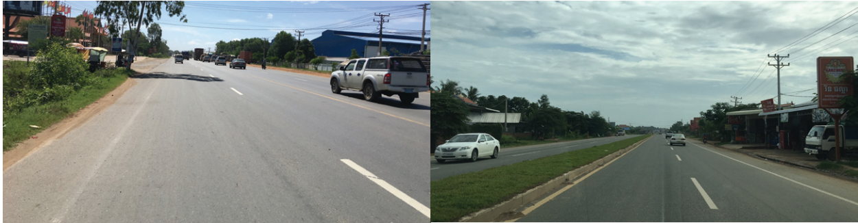
Left: Thnol Toteung–Phnom Penh . Four lane highway with asphalt concrete. Right: Phnom Penh–Skun . Four lane highway with asphalt concrete.
