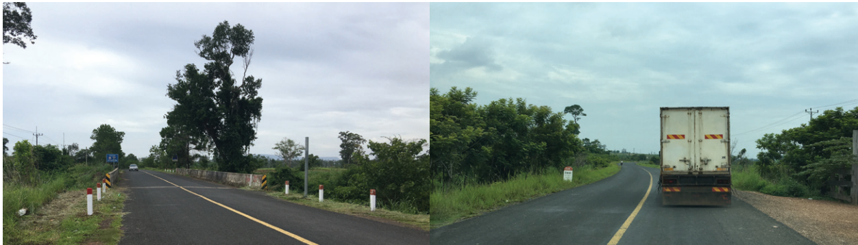
Left: Koh Keh–Tbeng Meanchey: Part of the 53 km road from Koh Ke to Tbeng Meanchey. Right: Tbeng Meanchey–Stung Treng: The road was rehabilitated in 2008 with double bituminous surface treatment surfacing.
