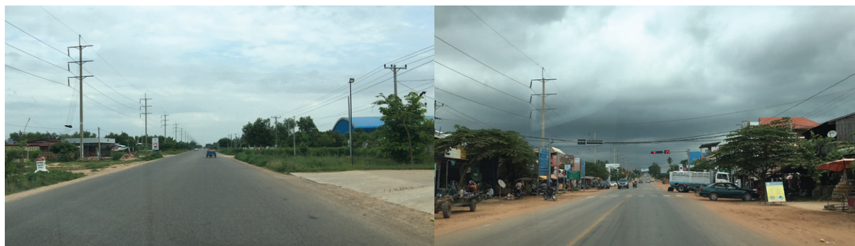
Left and right photos: Sections of Sisophon–Siem Reap. Asphalt concrete road was completed in 2008.
