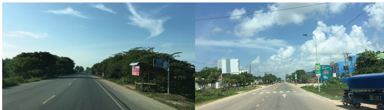
Left: Phnom Penh–Neak Leung . Existing condition of asphalt concrete road. Right: Neak Leung–Bavet Border . Double bituminous surface treatment road before resurfacing by asphalt concrete under an ADB loan.
