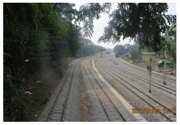
Note: Pre Final inspection for track profile are completed and Final manual rectification to close out the Track Geometry (Level and Alignment) are in progress.
