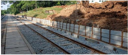
Lagging wall Panel installation was 100% completed.
