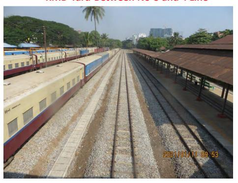
Note: Pre Final inspection for track profile are completed and Final manual rectification to close out the Track Geometry (Level and Alignment) are in progress.
